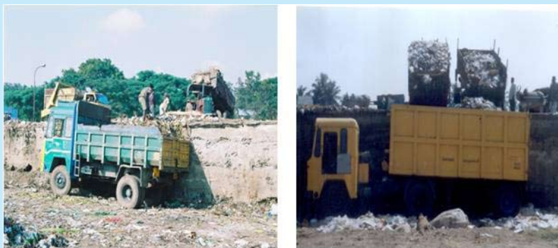
Figure 2.25: Site before commencement of work
