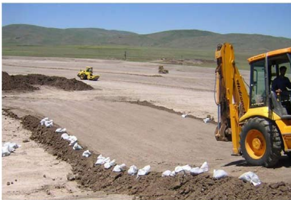
Figure 4.13: Construction of Test Field
