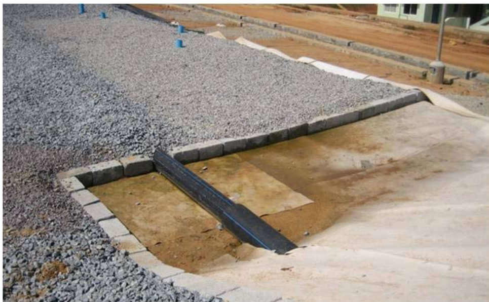
Figure 4.14: Test Field with all Sealing Components
