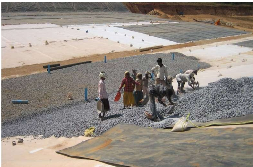
Figure 4.12: Sanitary Landfill under Construction
