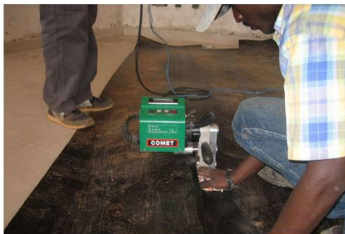
Figure 4.15: Welding of HDPE Geomembrane
