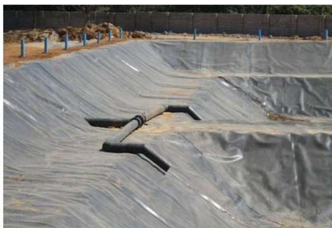
Figure 4.10: Sealed Leachate Pond with Two Basins
