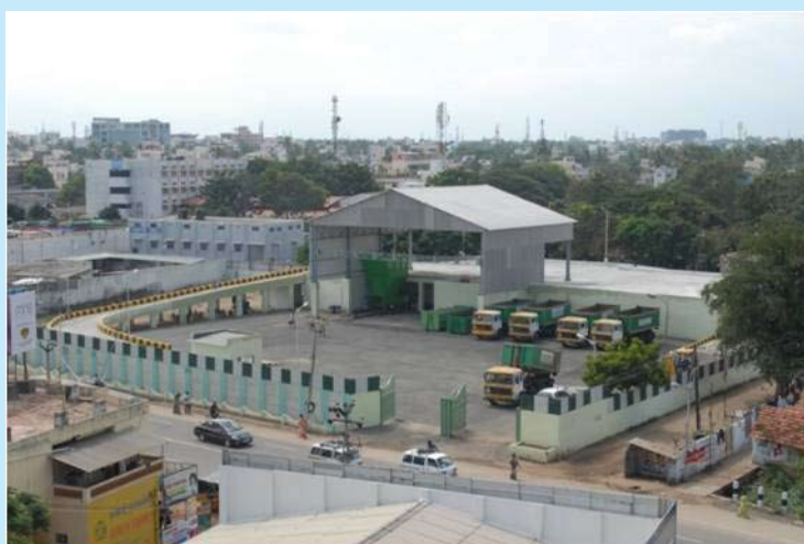
Figure 2.26: Site after commencement of work
