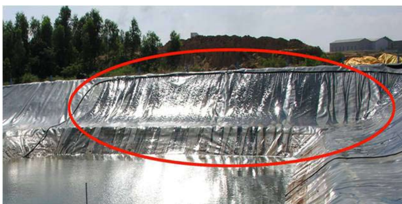
Figure 4.11: Irrigation of Leachate on the Slopes of the Pond
